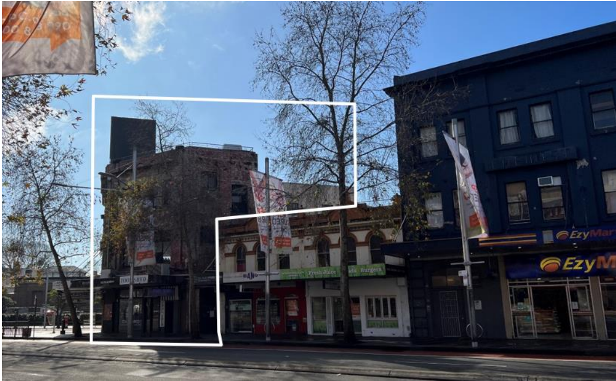
Figure 5: Site viewed from Flinders Street, and neighbouring buildings to the south
