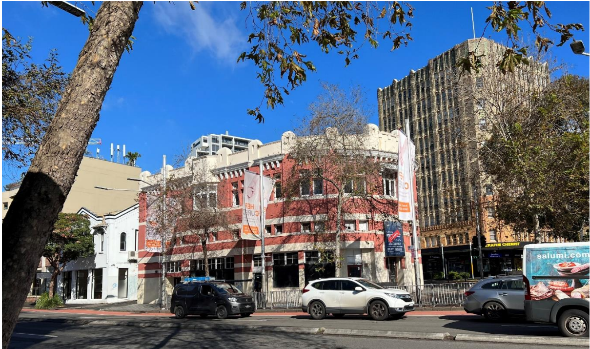
Figure 9: The 'T2' building (foreground) and the 'Belgenny' apartments (background) to the southeast
