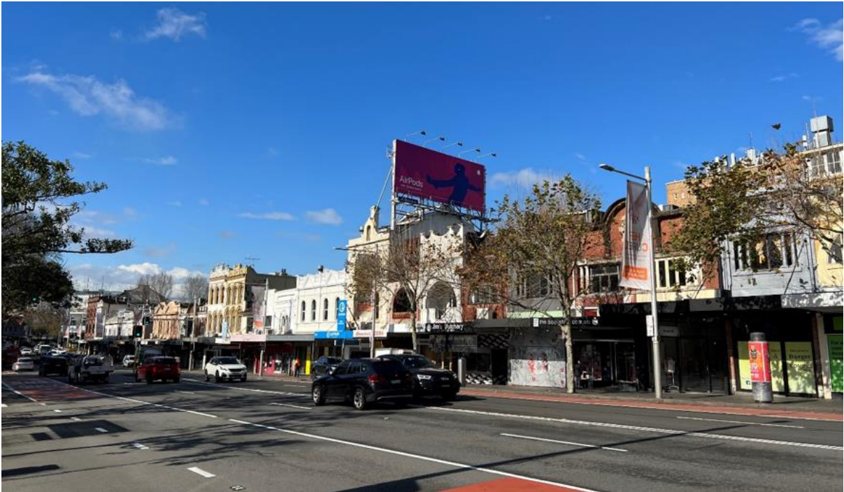
Figure 7: Neighbouring terraces to the east along Oxford Street
